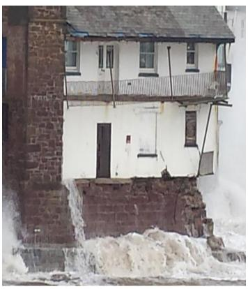
Serious damage by far was sustained by the Institute which was left in a very critical state. A hole had been punched in the east wall, and the outer wall supporting the lower balcony, and the balcony itself washed away leaving the base of the clock tower and the basement completely exposed.
